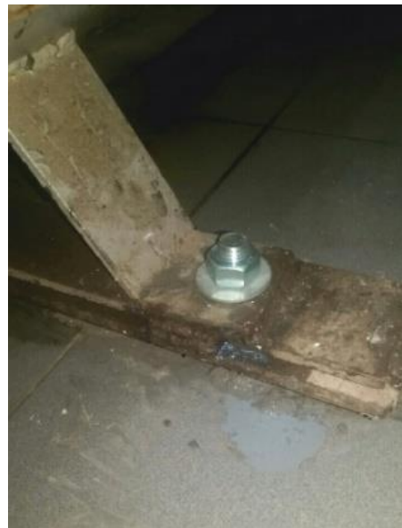
Fig. 5. Installation of anchor bolt in a borehole filled with acrylic composition
